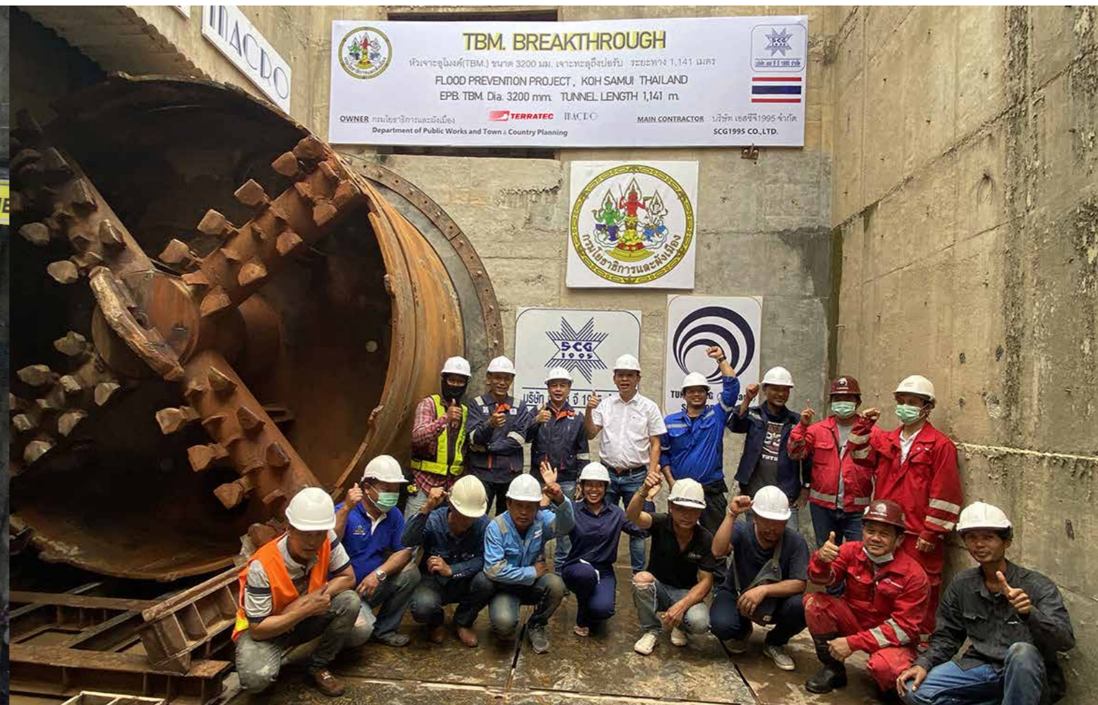
Thai contractor SCG (1995) Co Ltd. uses TERRATEC S48C refurbished Earth Pressure Balance Tunnel Boring Machine (EPBM) to excavate a 1.1km tunnel for the Samui Island flood control system.
