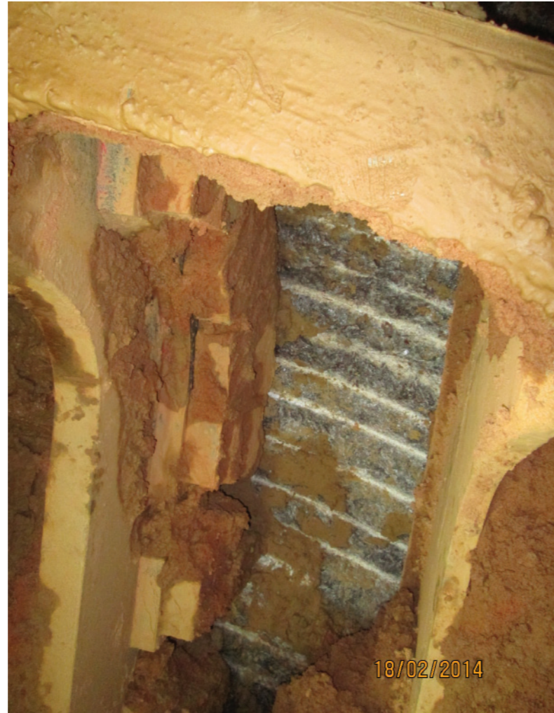
Project CC-07: Picture from inside of the TBM CutterHead showing the very hard quartzite.
