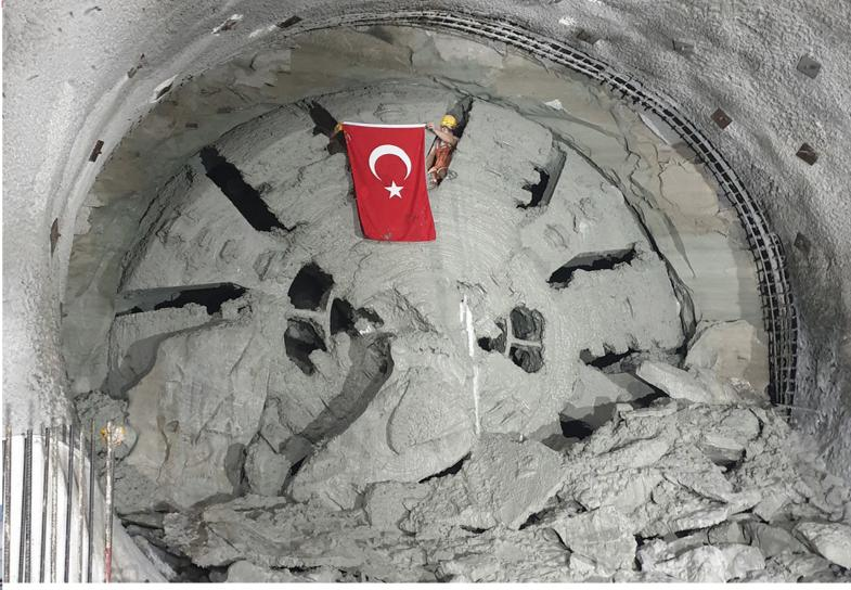
TERRATEC is pleased to announce that the first of four new 6.56m diameter Earth Pressure Balance Tunnel Boring Machines (EPBMs) currently working on the Ümraniye-Ataşehir-Göztepe (UAG) Metro line – which is being constructed by the Gulermak, Nurol & Makyol JV – successfully completed its first intermediate breakthrough on 20 May, into Atasehir Station.
