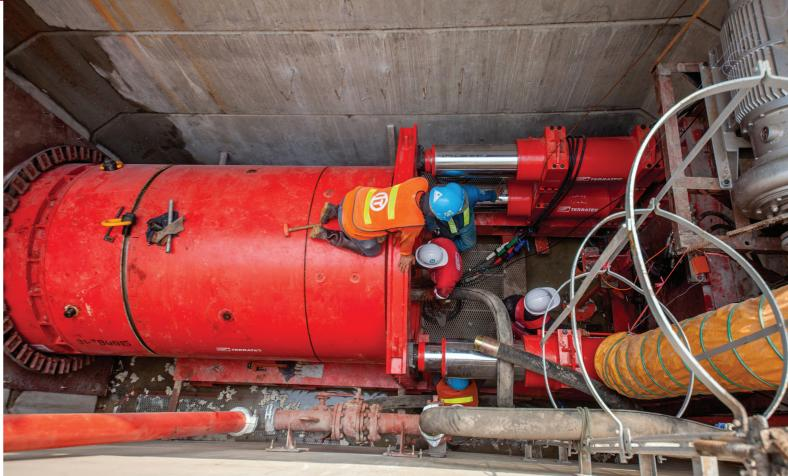
the assistance of Intermediate Jacking Stations. To date these MTBMs have been averaging 206m per month, and with 6,856m (79%) of the tunnelling works now complete on the project, progress is currently an impressive 40 percent ahead of schedule.
