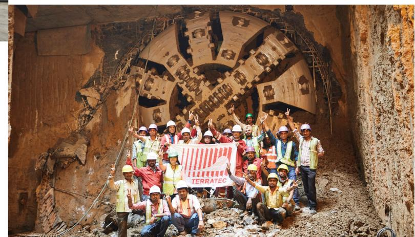
Two 6.61m diameter mixed/ rock EPB shields – S23 and S24 were deployed on Contract CC-07, part of the Violet Line (Line 6) Extension, by a joint venture of Russia's Metrostroy and local firm ERA Infrastructure.
