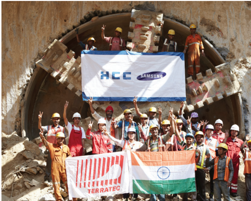
JV's Breakthrough Ceremony of S37 TBM in CC-34 Project
