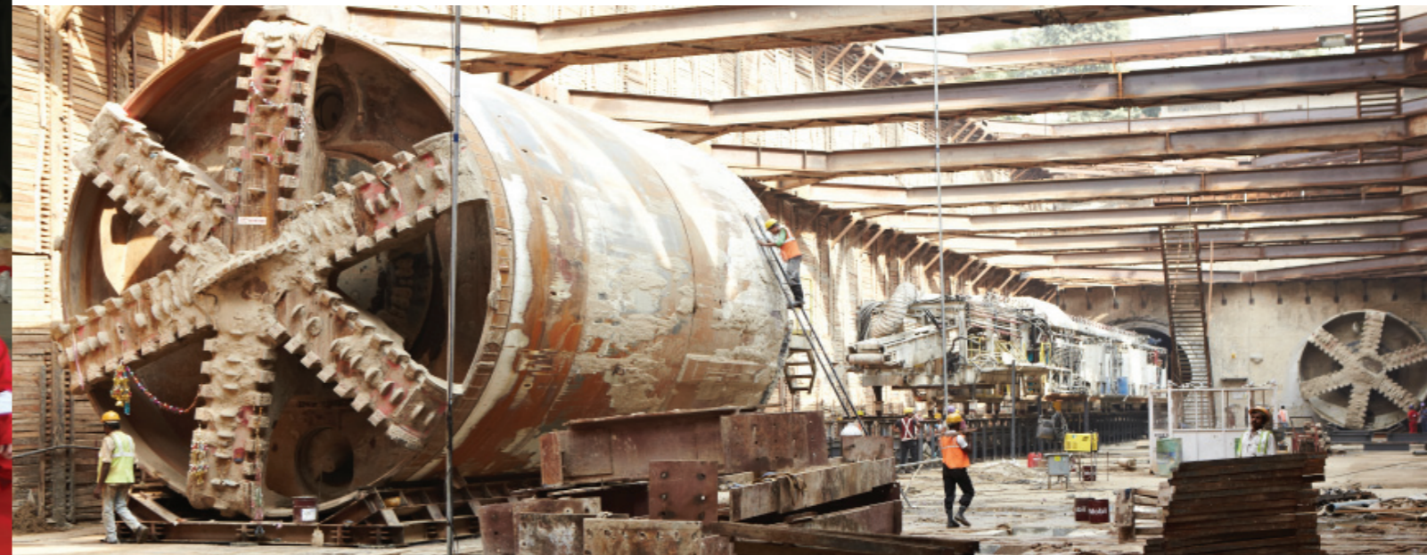
TERRATEC's S36 and S37 TBMs after breakthrough in CC-34 Project
